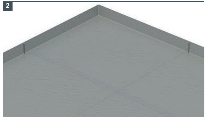
2 Measure the distances to the walls and edges. Set up the string line following the joint location.
