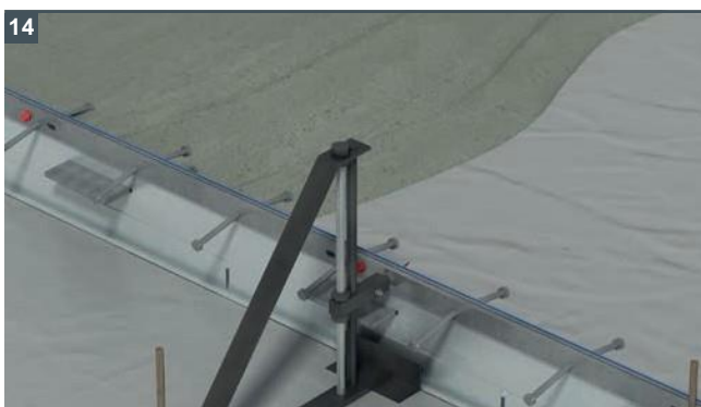
14 Pour the concrete while checking the height and position of the joint.
