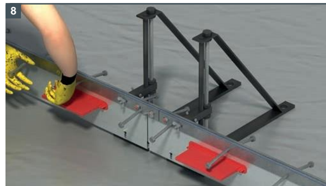
8 Manually position ArmourJoints in line with string lines.
