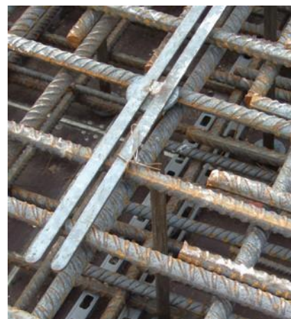
'Top down' installation. Rail is tied to the main reinforcement
